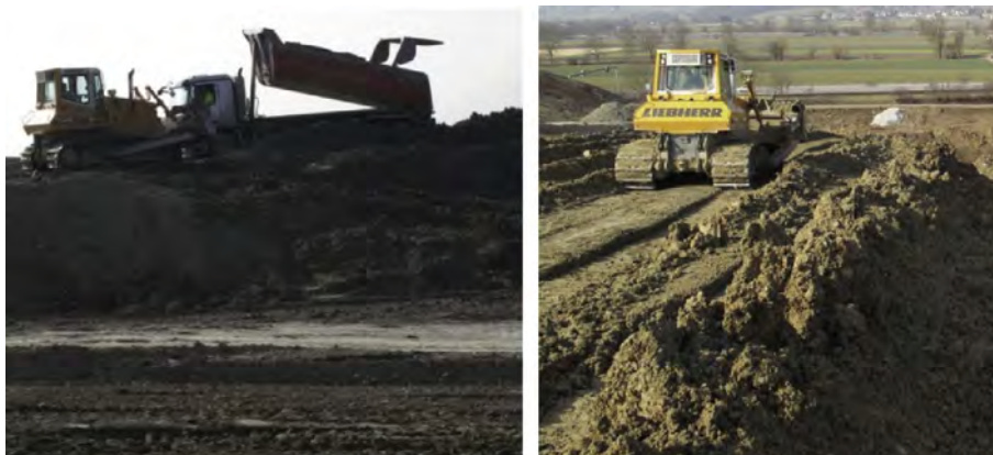
Fig. 9. Disposal of conditioned soil with favorable consistency.
